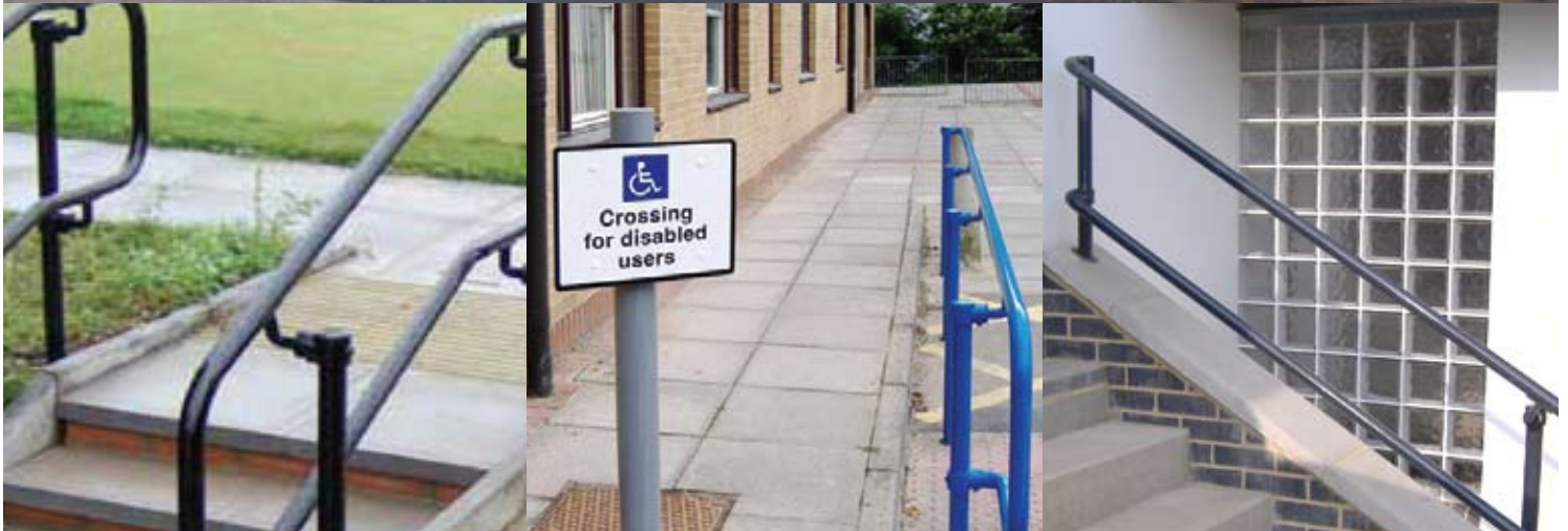
Mid rail comprises standard Kee Klamp® fittings
